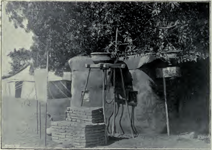
DEVELOPING HUT, TALNI CAMP.
